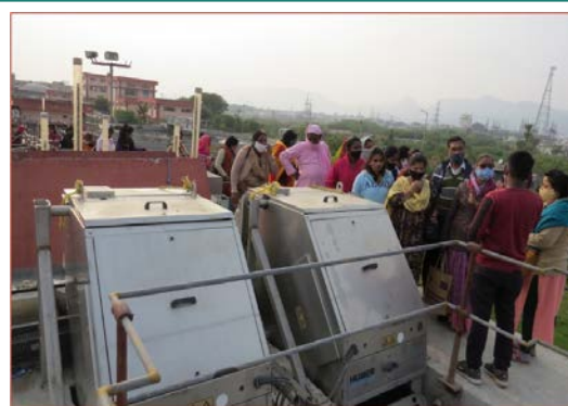
Participants during the site visit at Khanpura, STP, Ajmer, Rajasthan.
